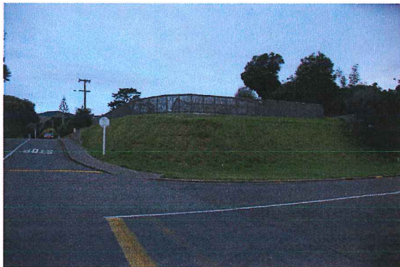
View from intersection of Renown and Tiromoana Roads
