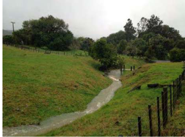
Figure 7: Existing drainage easement in proposed Lot 1 prior to being piped under ROW access
