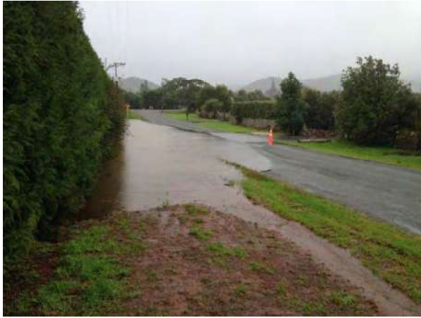
Figure 4: Surface water ponding and overtopping Golf Harbour Drive viewed north along carriageway
