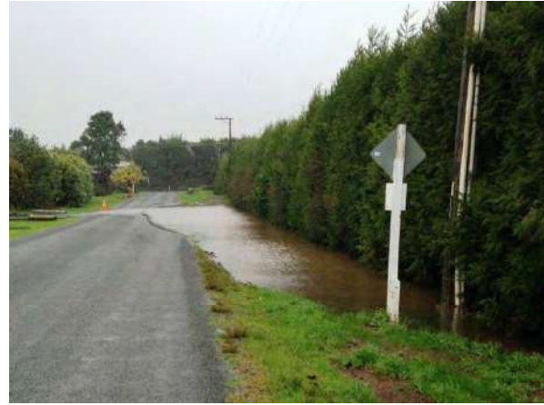
Figure 5: Surface water ponding and overtopping Golf Harbour Drive viewed south along carriageway
