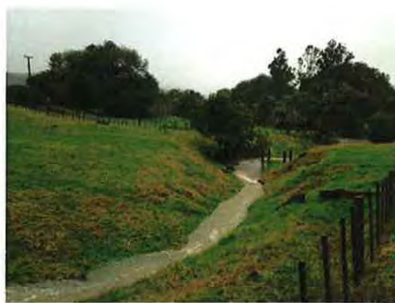
Figure 5: Existing drainage easement in proposed Lot 2 prior to being piped under ROW access
