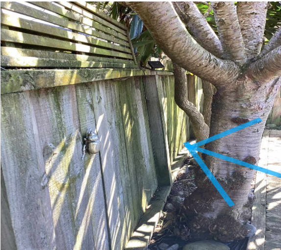
Fence leaning into neighbours property. This was noted to the rear boundary.
