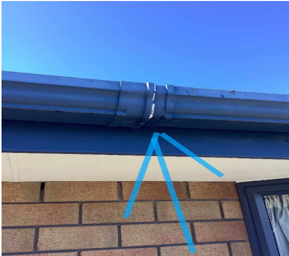
We recommend the leak is fixed to the guttering to the rear of the property as shown.
