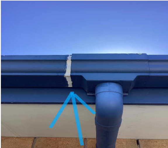
Left-hand elevation. The guttering has moved to the expansion gutter joiner.
