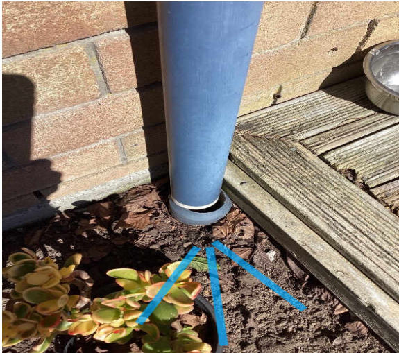
We recommend clipping downpipe back into outlet at ground level. This was noted to the right hand rear corner elevation.
