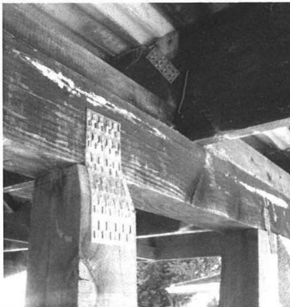
Photo 2. Roof beam/post connection
