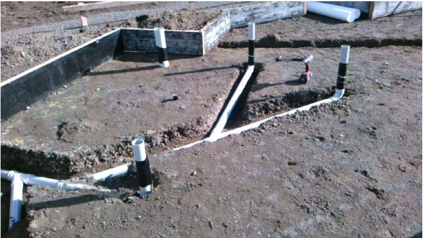
65mm wastes running to grey water gully Taken at 3:04 PM on Wednesday 22/08/2018
