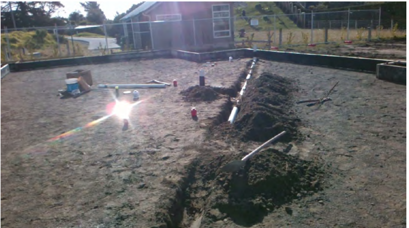
branch drain under the slab Taken at 3:04 PM on Wednesday 22/08/2018
