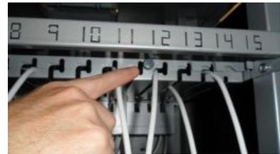
4. Remove the cables to be replaced by pulling them out of the cable management channel and unwinding from the cleat at the back of the shelf.
