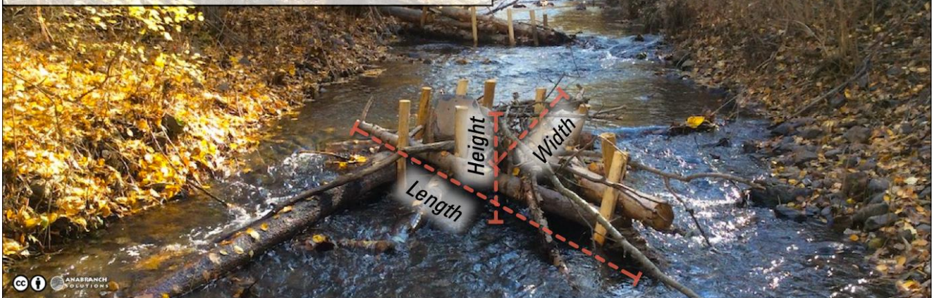
FIGURE 25. TYPICAL EXAMPLE OF A POST – ASSISTED LOG STRUCTURES (PALS) SHOWING STRUCTURE DIMENSIONS USED IN STRUCTURE SPECIFICATION
