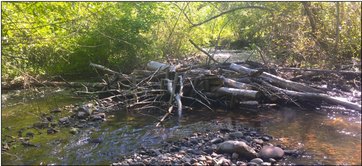
Figure 11. Example of a mid-channel post-assisted log structure (PALS) designed to mimic woody debris accumulations.
