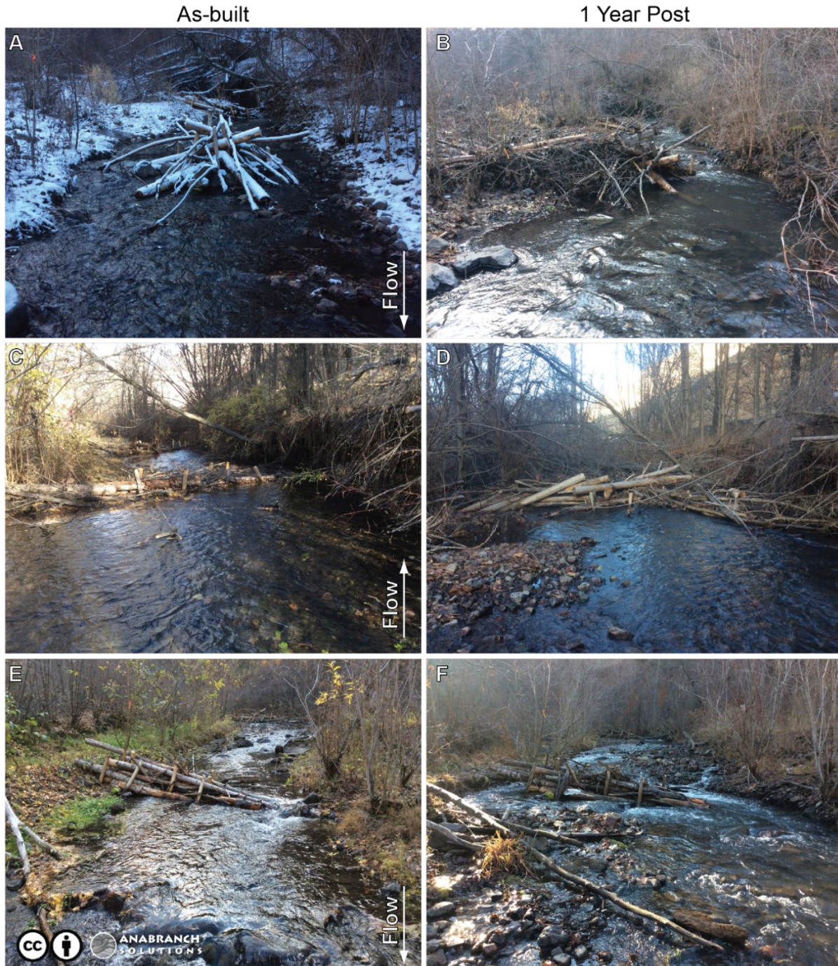
Figure 23. Example of PALS evolution over the course of one year promoting processes of wood accumulation. A and B show a mid-channel PALS becoming a bank-attached PALS, C and D show a bank-attached PALS becoming a debris jam, and E and F show a bank-attached PALS becoming a mid-channel PALS. The geomorphic changes imposed by the presence of the PALS in each example shows clear alterations to the channel bed and hydraulics. From Chapter 4 of Wheaton et al. (2019: http://lowtechpbr.restoration.usu.edu ).
