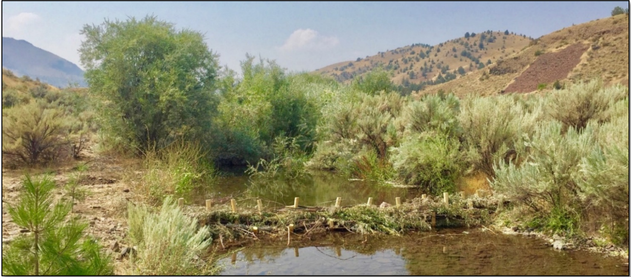
Figure 12. Example of beaver dam analogue (BDA) reinforced with posts.
