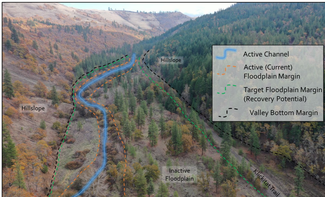
Figure 5. Conceptual schematic of valley bottom geomorphic composition in the lower Swale Creek project area. Note that the target floodplain is limited by the old railway prism running parallel to the valley bottom on the right side of the photo.
