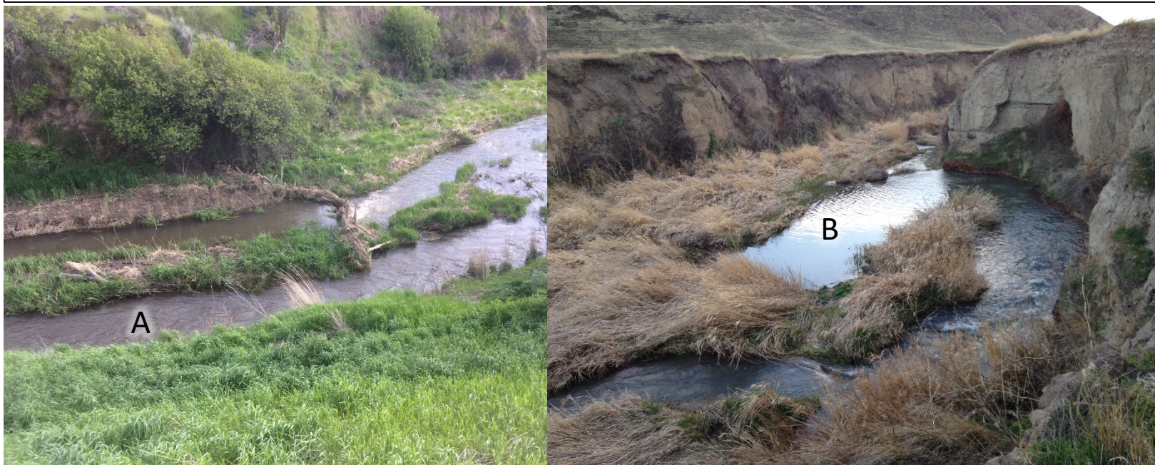
Figure 1. Two BDA structures on Pataha Creek during receding high flows. Note A) activated side channel and B) ponding upstream of BDA. Areas such as these were heavily planted with willow and cottonwood whips and poles to take advantage of increased water retention and fresh fine sediment deposits.
