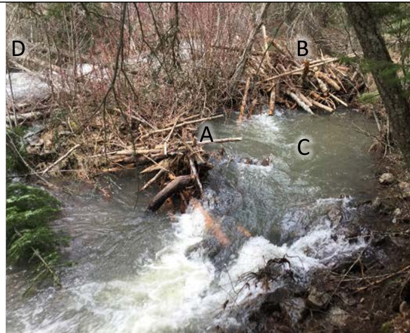
Figure 1. Pre (Feb. 2017; left photo) and post (March 2017; right photo) high flow images of PALS 48. In the post high flow photo, note A) debris accumulation on the original PALS, B) debris from failed upstream PALS on the upstream large wood spanner, C) pool formed upstream of structure/downstream of debris jam, and D) activated side channel in the far background.
