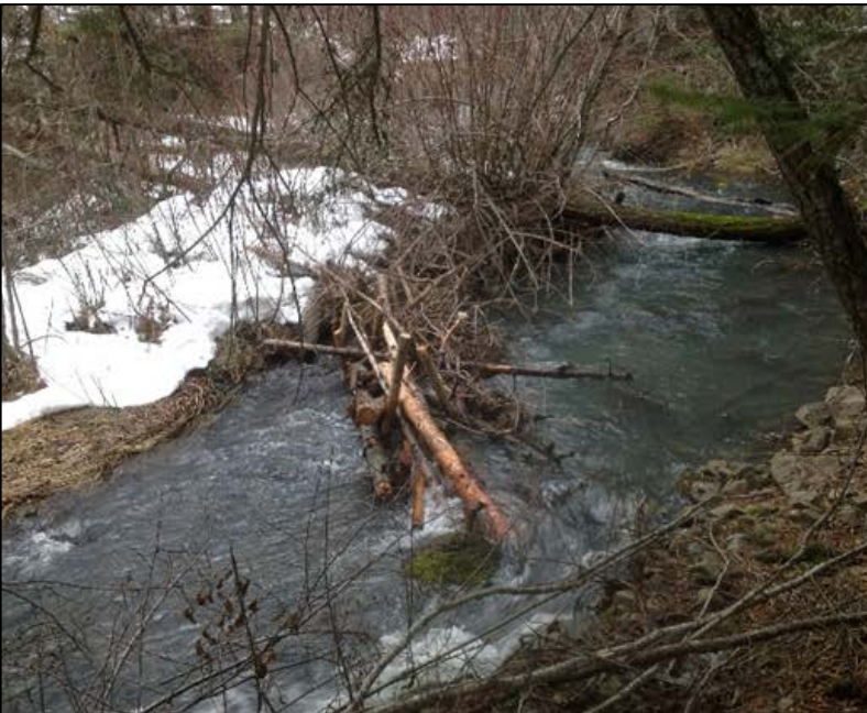
Figure 1. Pre (Feb. 2017; left photo) and post (March 2017; right photo) high flow images of PALS 48. In the post high flow photo, note A) debris accumulation on the original PALS, B) debris from failed upstream PALS on the upstream large wood spanner, C) pool formed upstream of structure/downstream of debris jam, and D) activated side channel in the far background.
