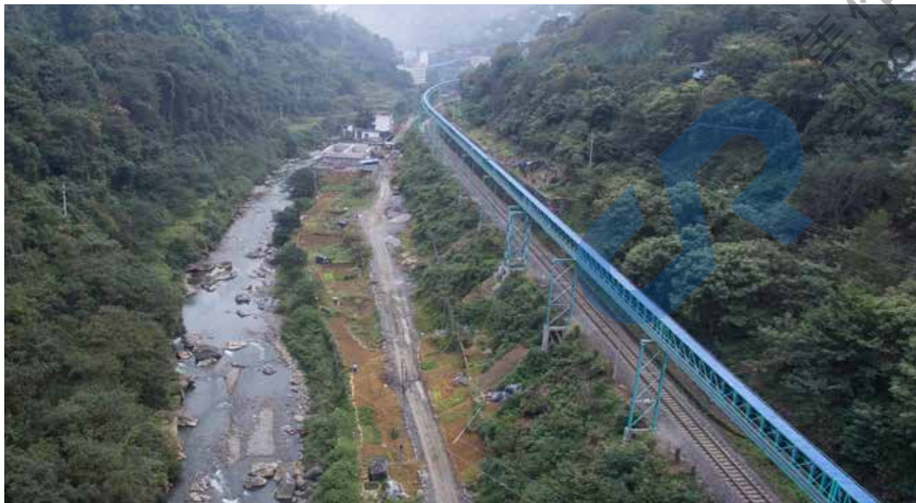
安稳管带机 Pipe conveyor for Anwen Power Plant
