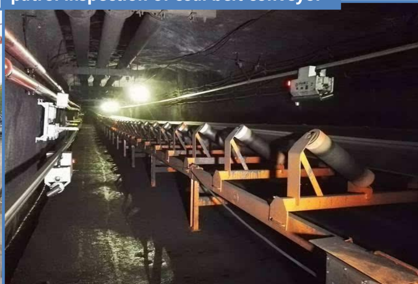
patrol inspection of coal belt conveyor
