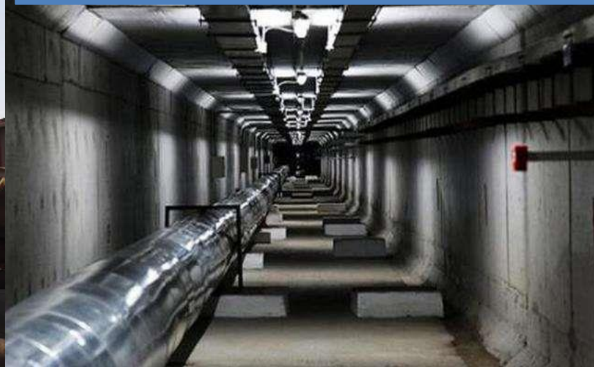
corridor inspection of municipal pipe
