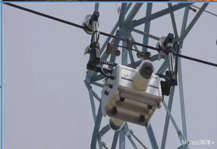
line inspection of overhead transmission
