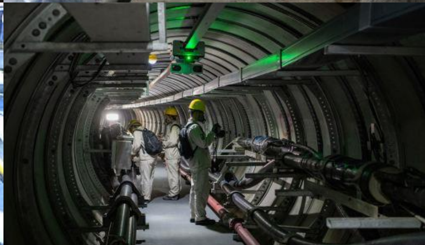
cable tunnel inspection
