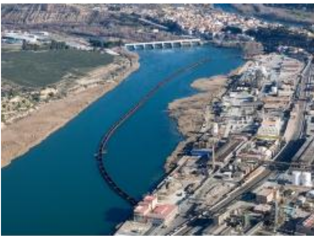
Figure 8 Water reservoir in Flix. Note barrier to impede mixture and spreading of the chemical waste.
