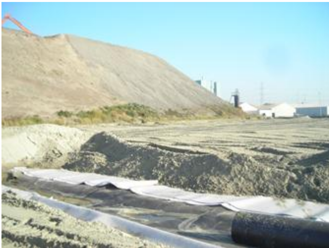
Figure 10 New cell of landfill in Belgium
