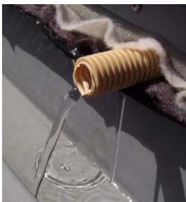
Figure 5 Combination of a draining blanket with mini-pipes
