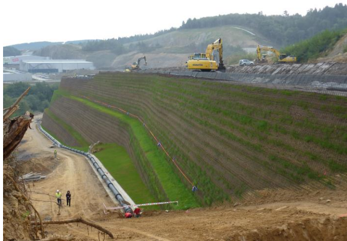
Figure 7 Green wall forming a 30 m high reinforced embankment in Bilbao, Spain
