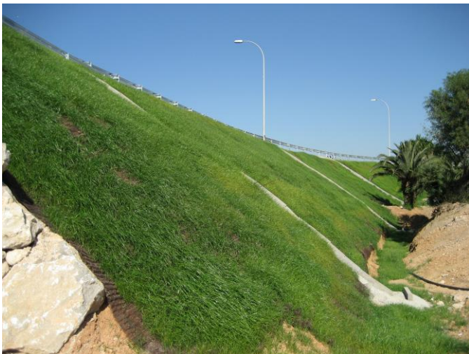
Figura16 Fully vegetated soil with volumetric erosion control geocomposite
