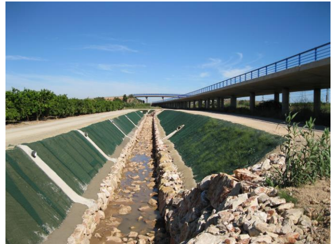
Figure 14. Slopes covered with the volumetric erosion control geocomposite
