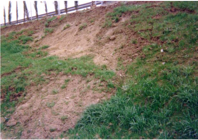
Figure 1 Erosive process in a slope
