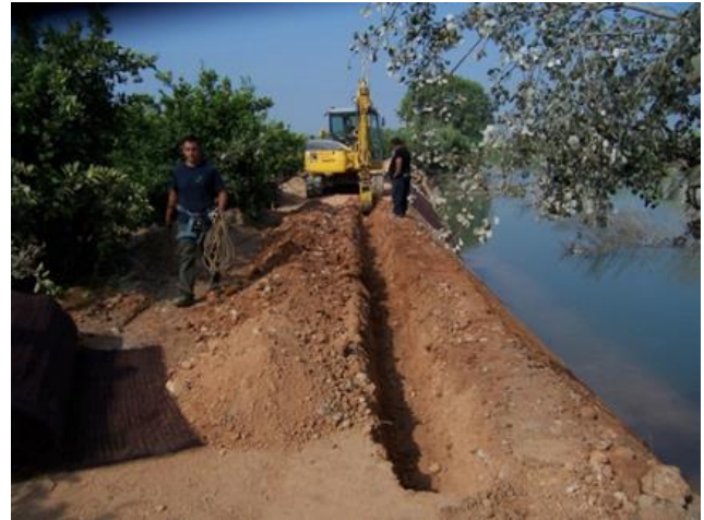
Figure 6 Excavation of the anchor trench
