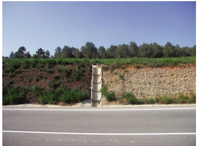
Figure 10 Slope with and without volumetric erosion control geocomposite
