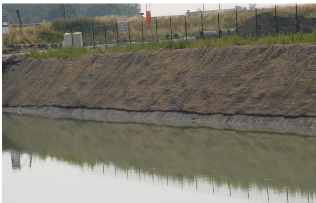
Figure 12 Reservoir with volumetric erosion control product
