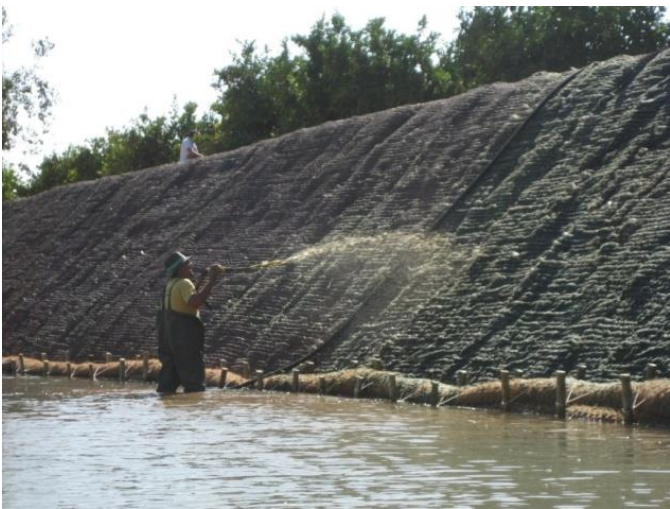
Figure 9 Hydroseeding
