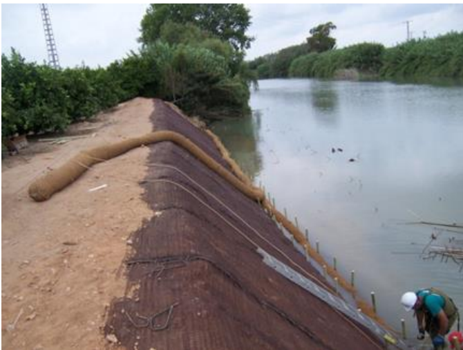
Figure 8 Installation process: Ensuring a proper anchorage
