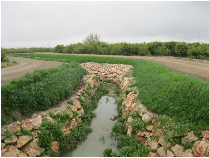
Figure 15 Fully vegetated channels
