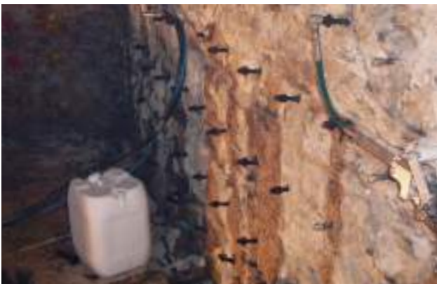
Positioning of packers on natural stone masonry
