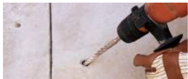
Positioning of drill holes for sealing expansion joints
