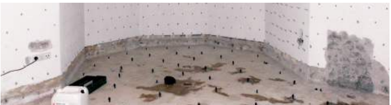
Positioning of packers on wall and floor surfaces
