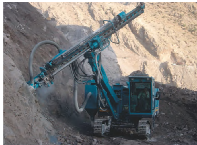
伊朗施工 Construction in Iran
