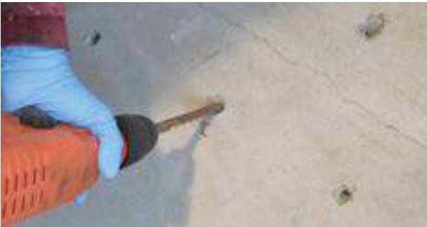
Ill. 1: Making drill holes
