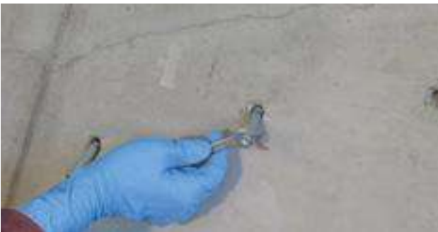
Ill. 3: Tightening packers
