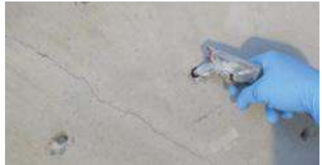
Ill. 2: Removing drill dust
