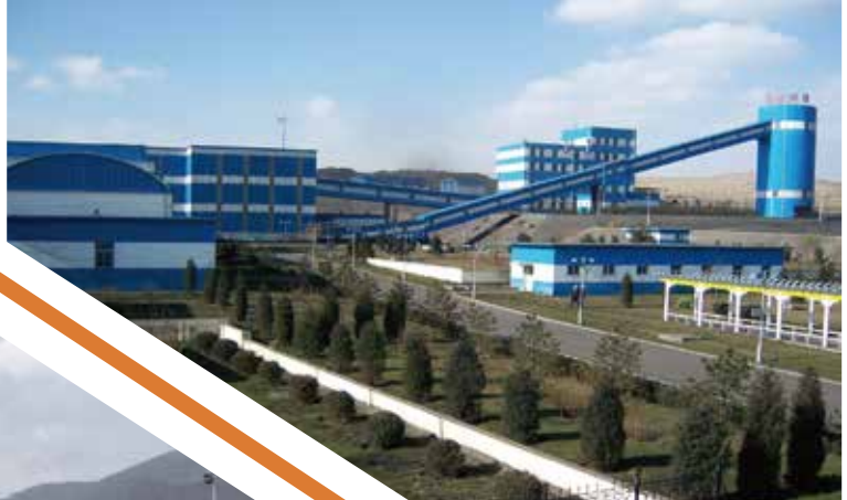
Sichuan Dazhou Coal Handling Plant Belt Conveyor for Coal Handling Plant
