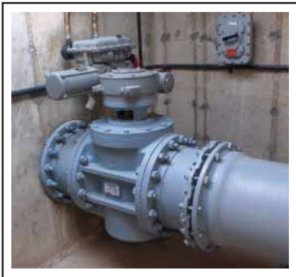
Cam-Centric® Plug Valve with motor actuator
