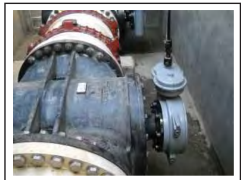
Cam-Centric® Plug Valve with worm gear actuator and extension stem
