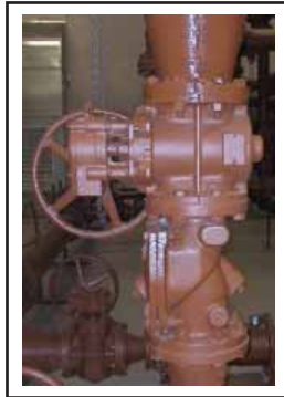
Cam-Centric® Plug Valve with Val-Matic Swing-Flex®
