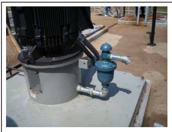
Air/Vacuum Valve with Dual Port Throttling Device
