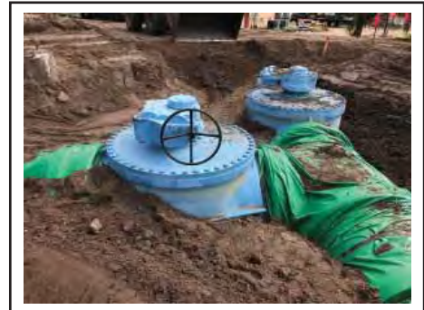
Cam-Centric® Plug Valve with worm gear actuator
