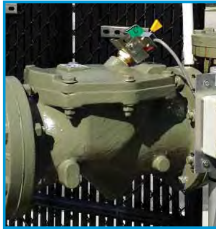
Swing-Flex® Check Valve with Limit Switch
