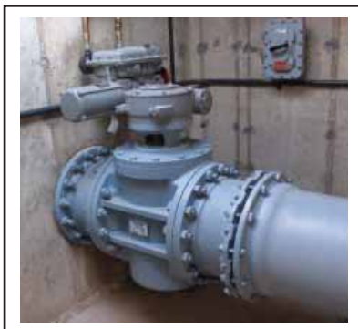
Cam-Centric® Plug Valve with motor actuator
