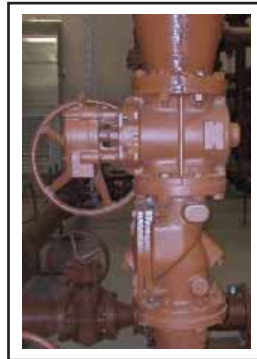
Cam-Centric® Plug Valve with Val-Matic Swing-Flex®
