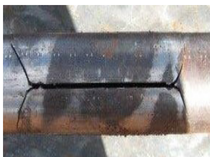
FATIGUE - T SHAPE DUE TO EXCESS CLAMP LOAD
