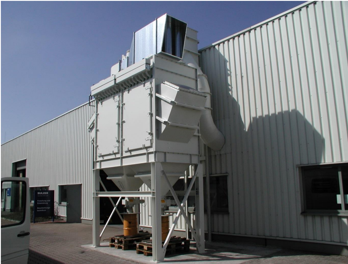
Compact filter unit for a thermal coating plant in Barchfeld, Germany Air flowrate: 15,000 m 3 /h, ATEX compliant explosion proofing
