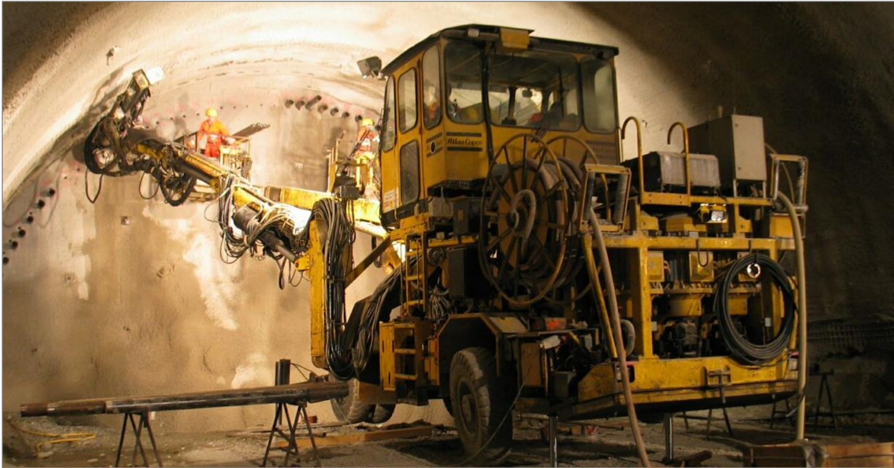
Example of a drilling rig
