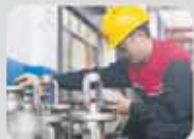
Wall thickness test
