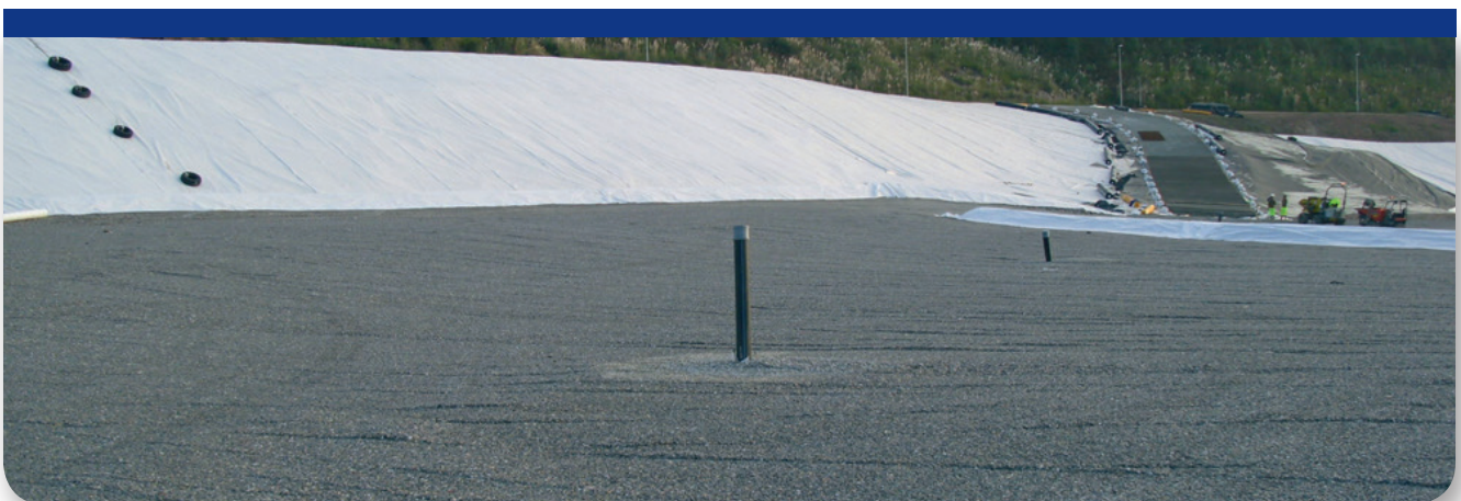
Fig. 10. Normalizing layer of gravels in the bottom of the landfill.
