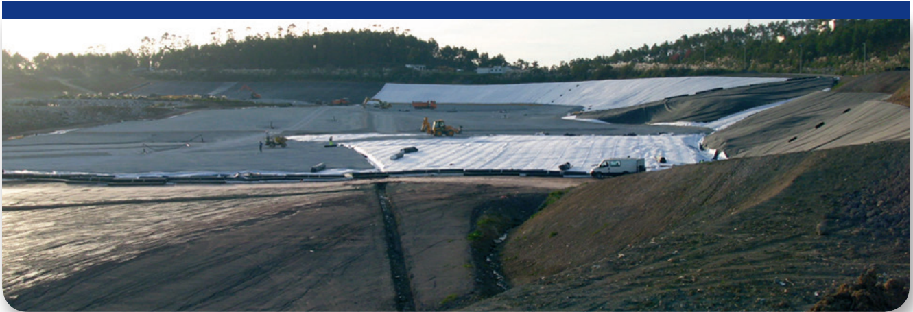
Fig. 9. General overview of Meruelo new cell under construction.
