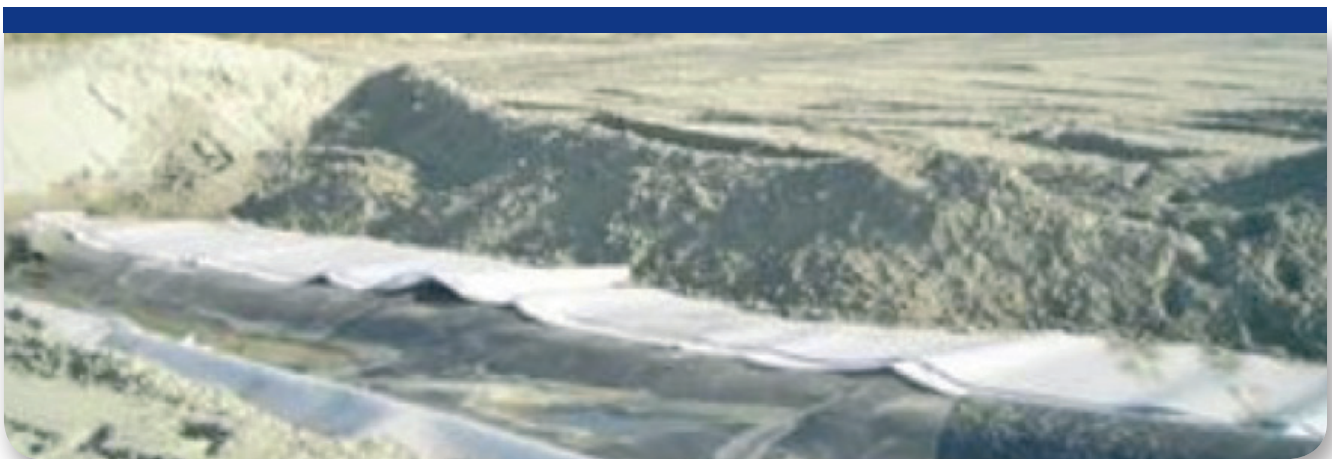
Fig. 6. Indaver landfill. The drainage composite is deployed directly over the geomembrane.
