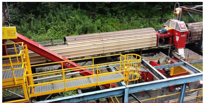
Two Stage Sampling System in Existing Structure
