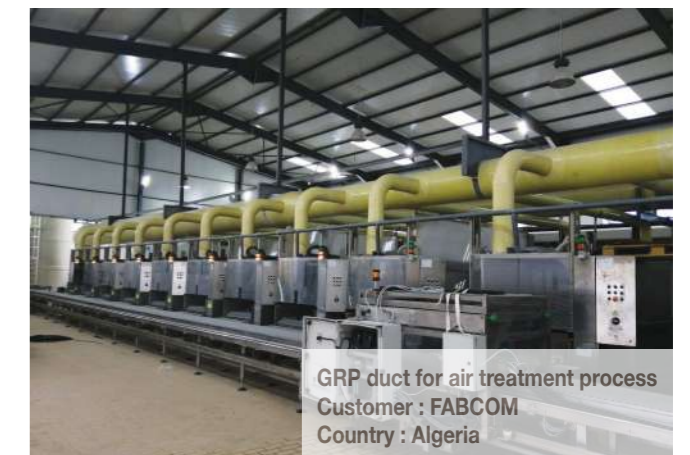
GRP duct for air treatment process Customer : FABCOM Country : Algeria
