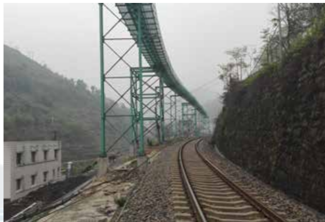
Anwen Power Plant , China
