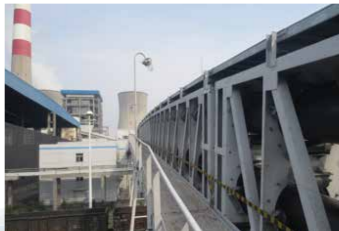
Kaifeng Power Plant , China
