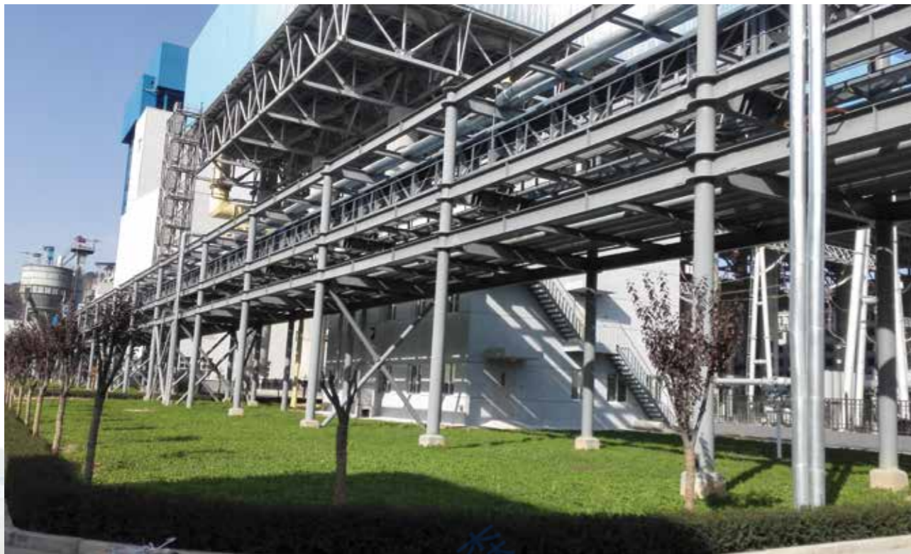
Huangling Power Plant , China
