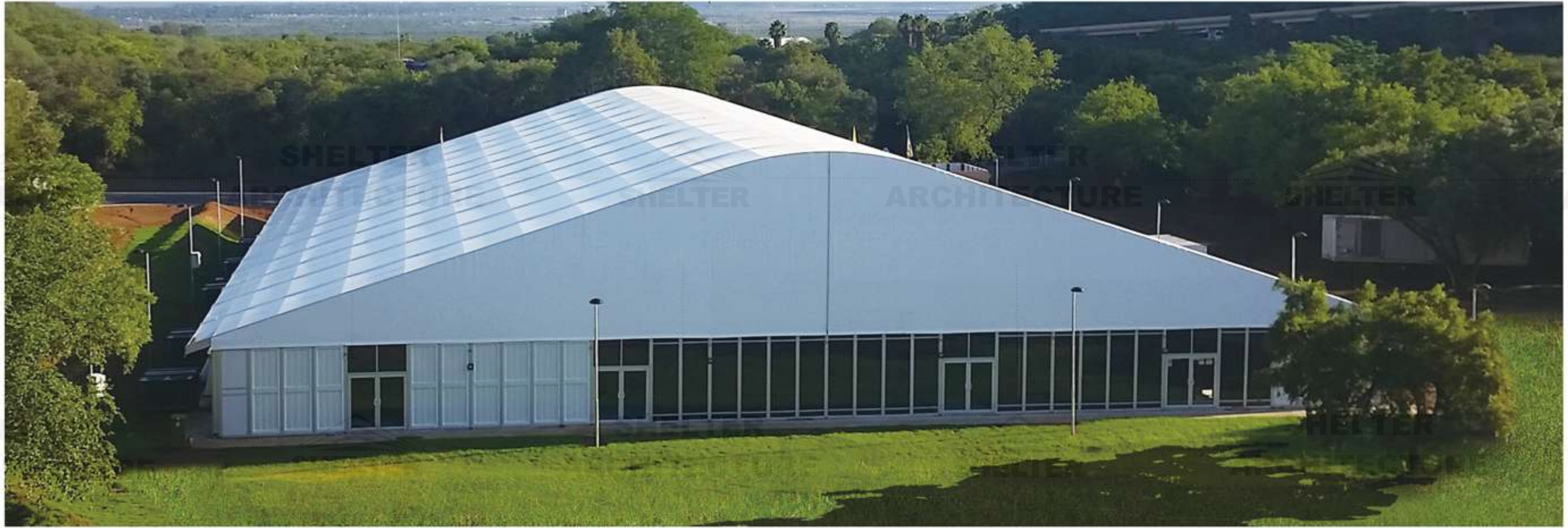
Storage Tents For Logistics Center South Africa
