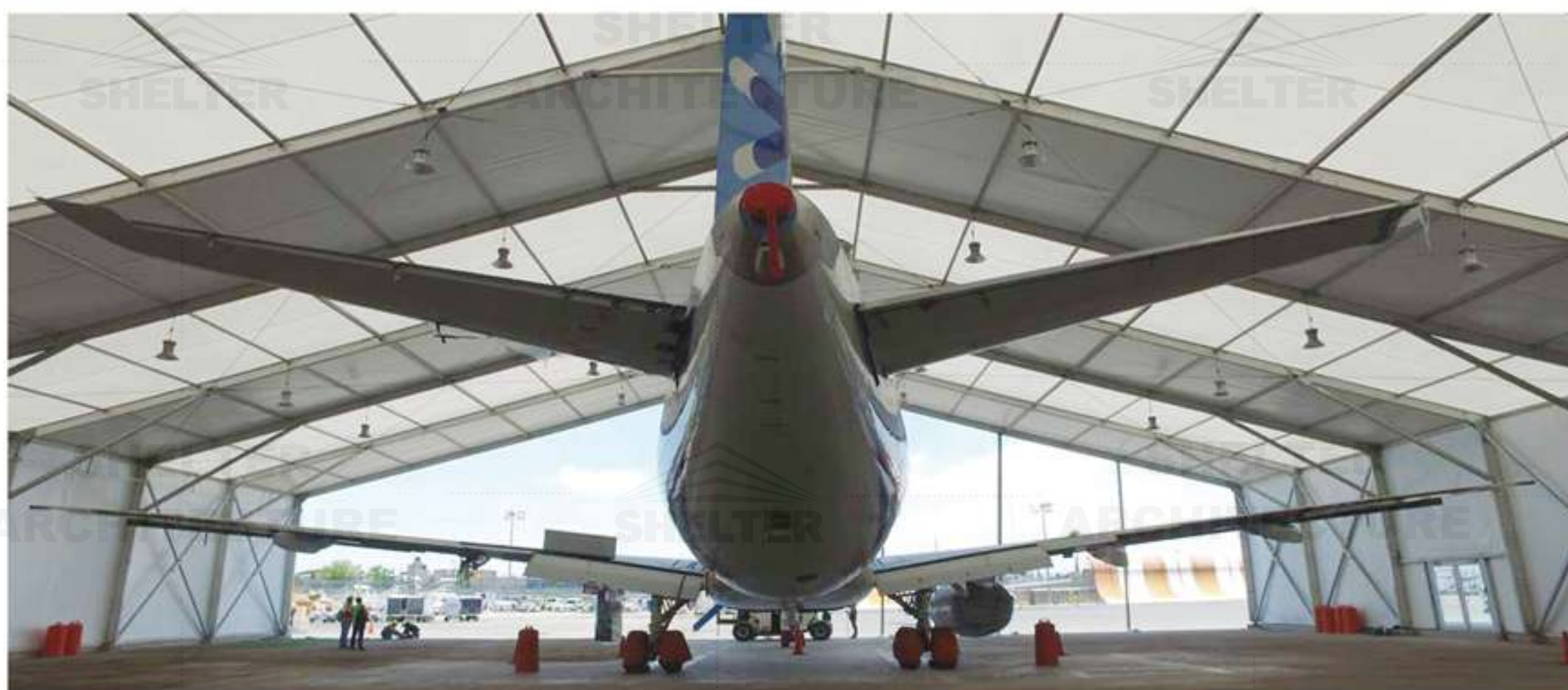
Aircraft Hangar for Ministry of Defense and Civil Aviation
