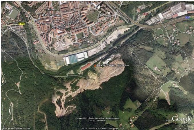
Photo No. 1 Aerial view of the work area
