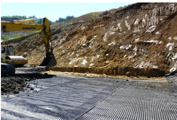
Photo No.4: Home Filler reinforced embankment
