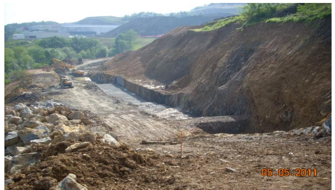
Photo No.6: Preparation of the support base
