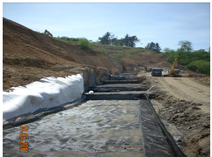
Photo No. 7 Start working with the first mesh of 300 kN.
