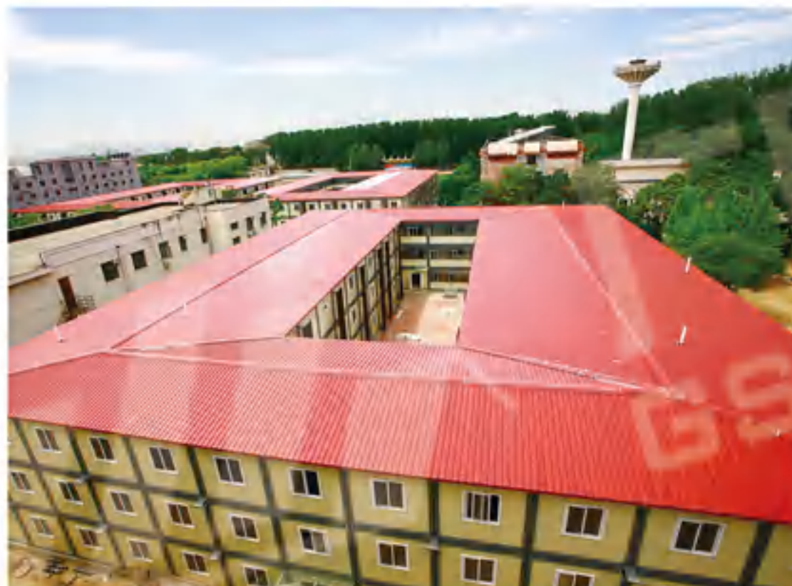
红色四坡屋顶 Red four slope roof
