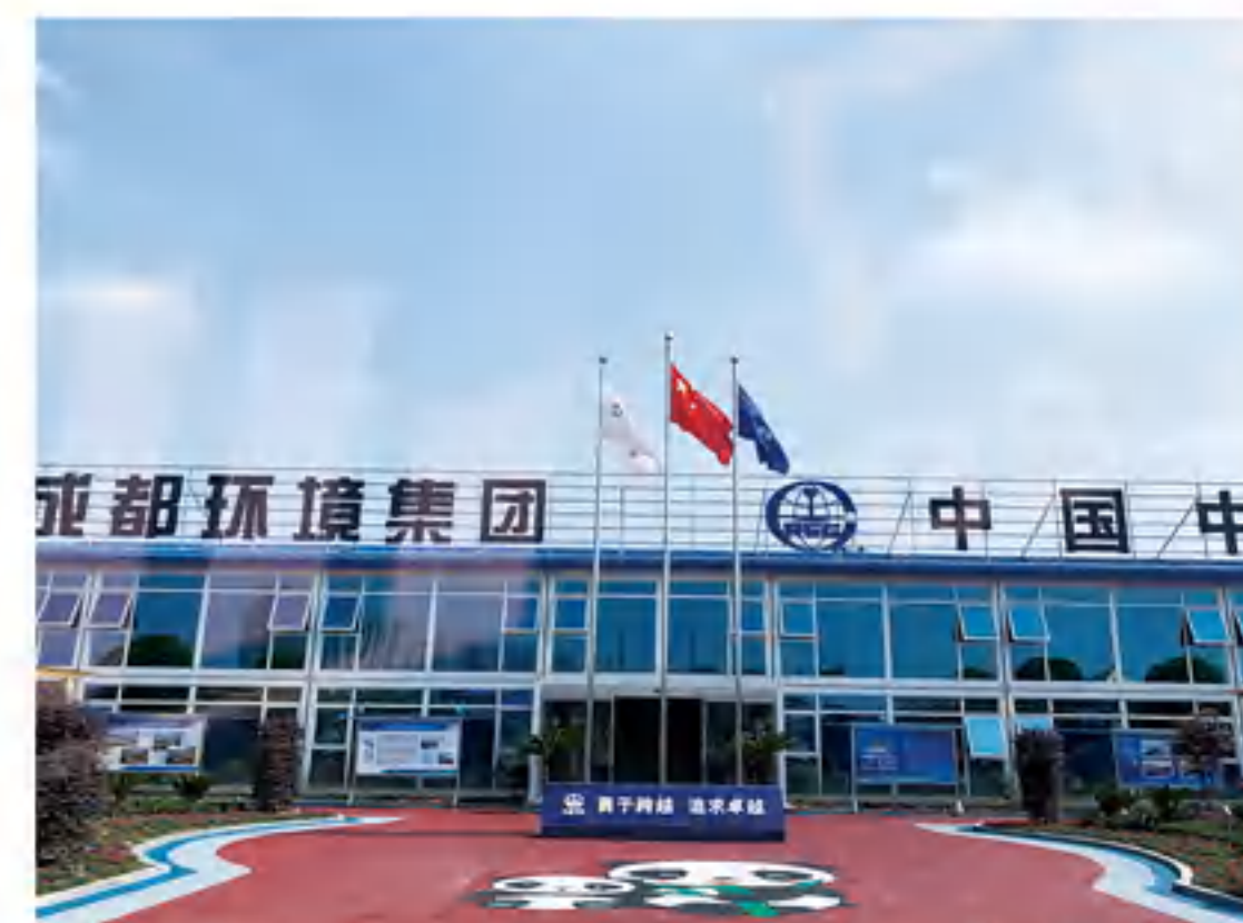
中铁上海工程局成都骑龙净水厂项目 REC Shanghai Engineering Bureau Chengdu Qilong Water Purification Plant Project
