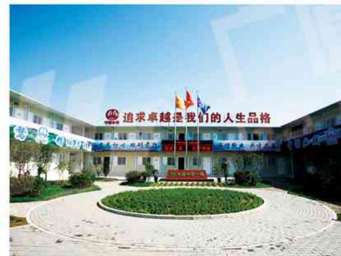
中铁一局雄安新区9号地一期造林项目 REC First Bureau Xiong'an New District No. 9 Afforestation Project
