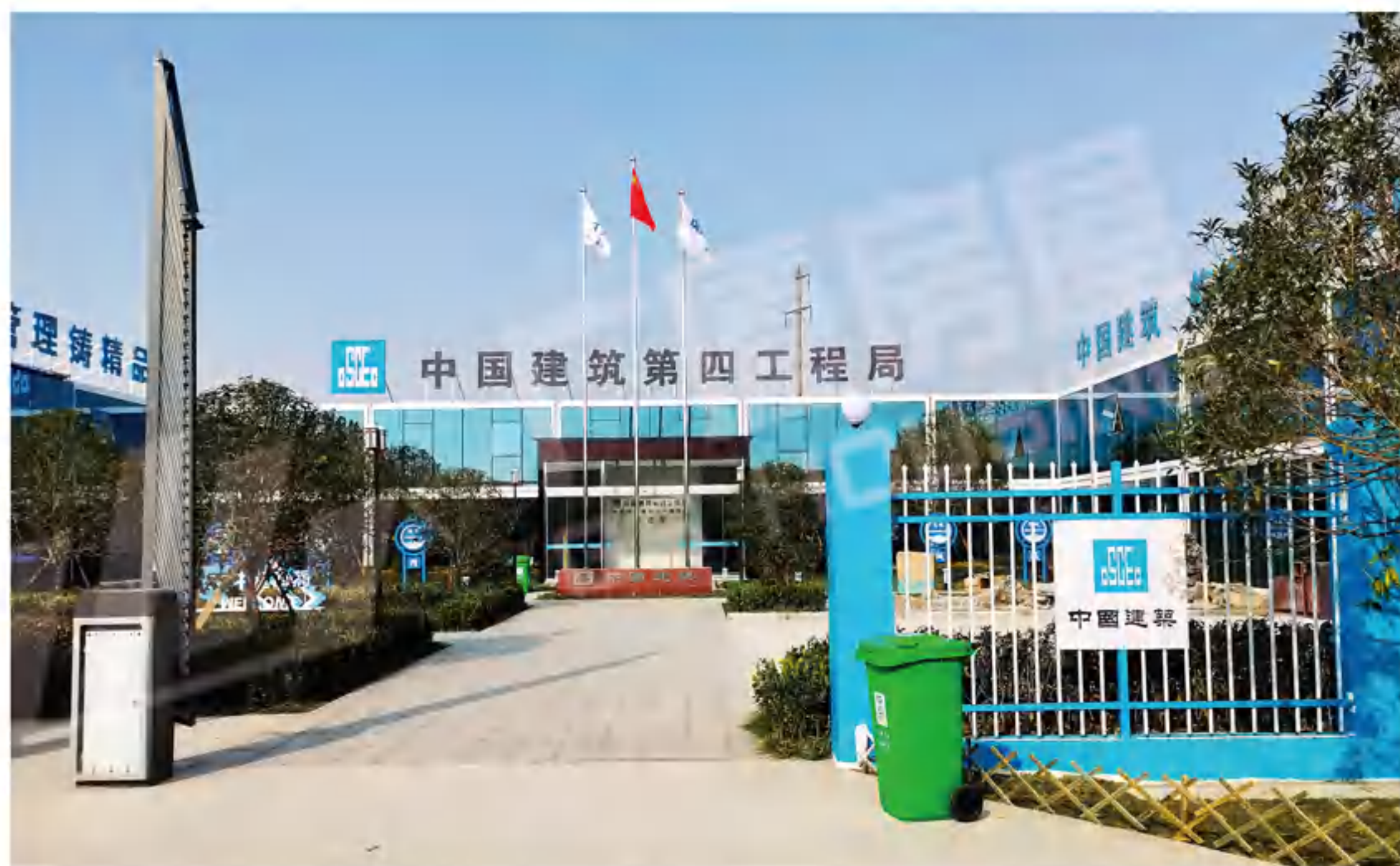
中建四局杭州会展中心项目 CSCEC 4th Bureau Hangzhou Conference and Exhibition Center Project
