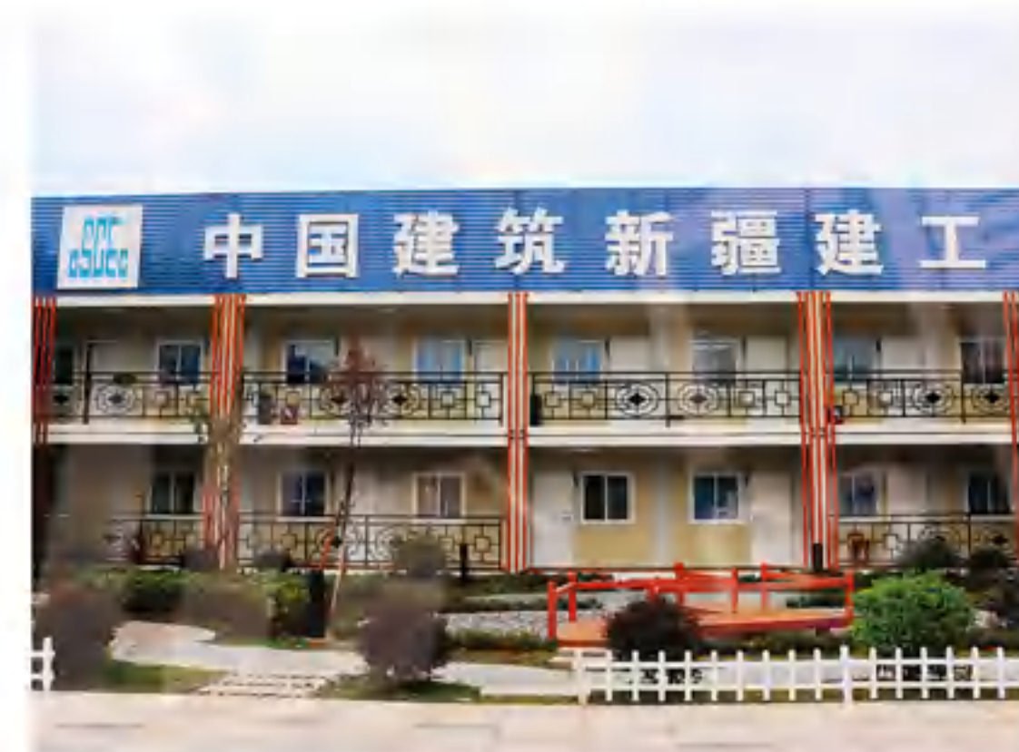
中建新疆建工广州龙城国际康复医院项目 CSCEC Xinjiang Construction Engineering Guangzhou Longcheng International Rehabilitation Hospital Project
