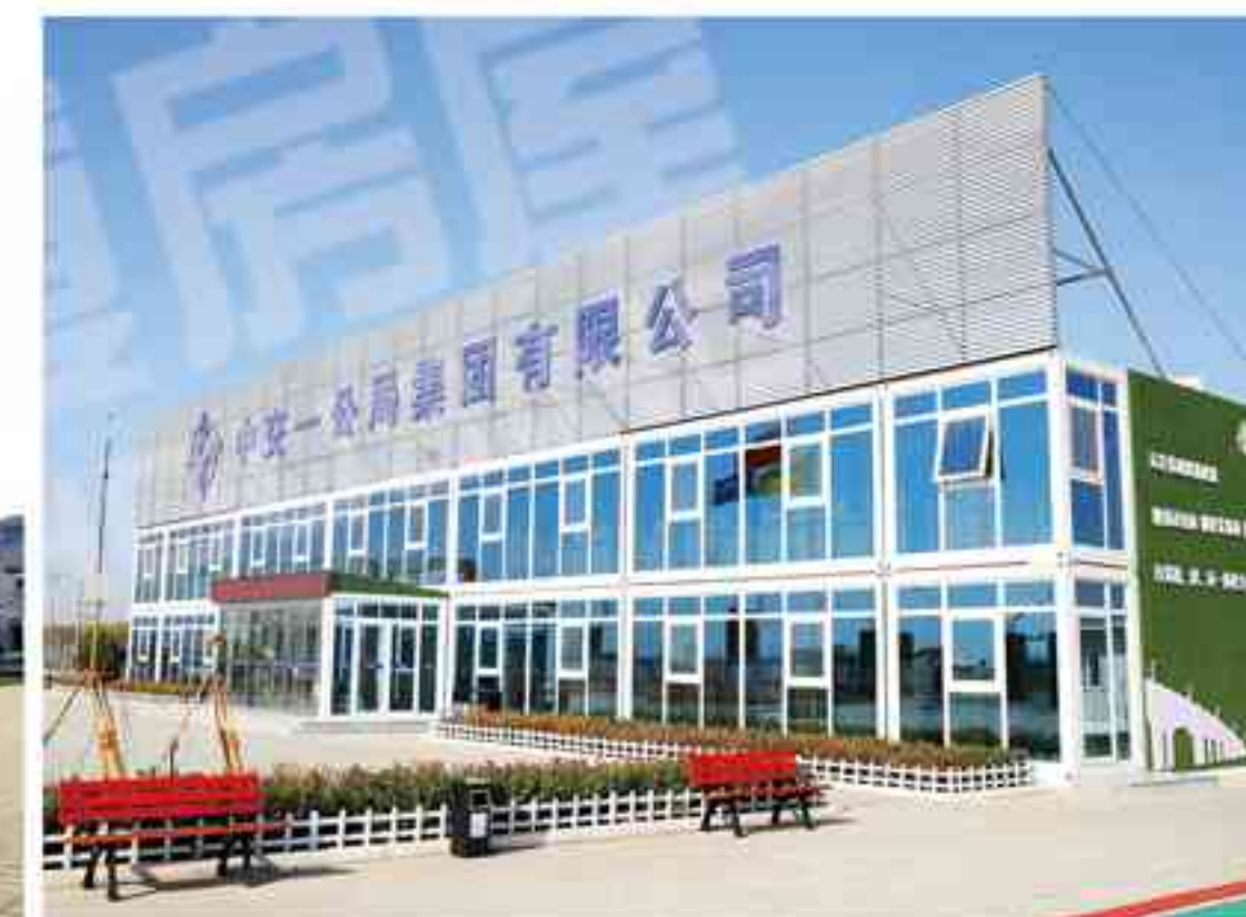
中交一公局雄安容东片区临时土方堆存项目 CCCC Temporary Earthwork Storage Project in Rongdong Area of Xiong'an
