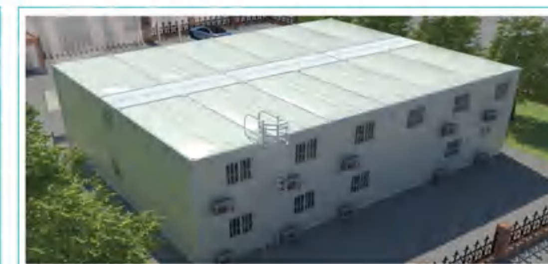
检修爬梯 Maintenance Ladder
