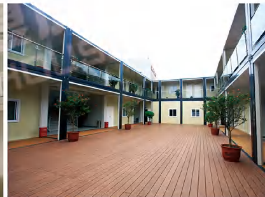
走廊箱+玻璃护栏 Corridor box + glass guardrail
