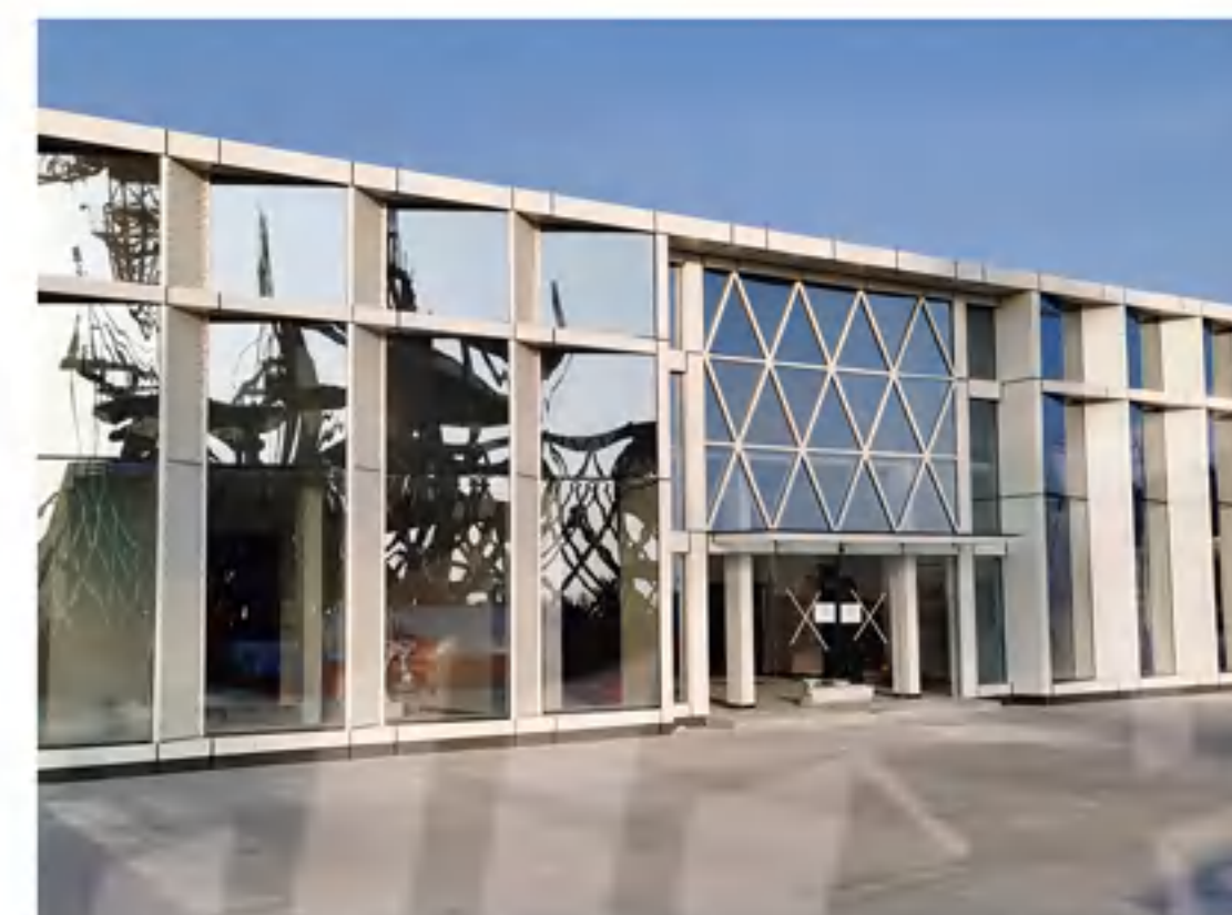
中建六局三亚崖州科创中心展馆 CSCEC 6th Bureau Yazhou Science and Technology Center Exhibition Hall
