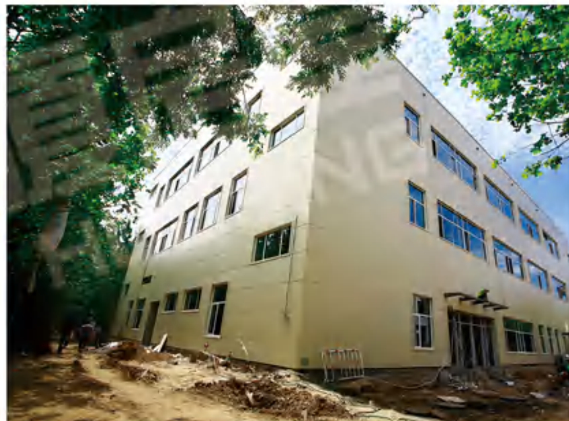
快装房多功能会议室 Multifunctional meeting room
