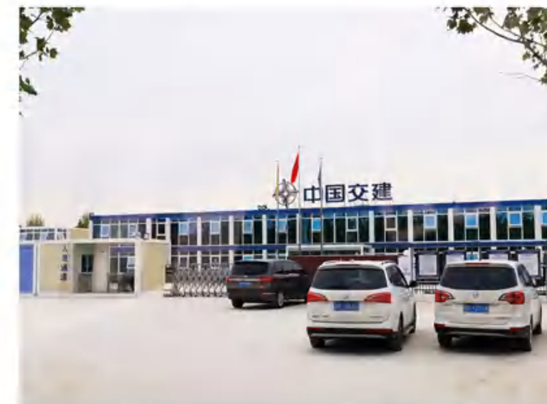
中交天航局菏泽黑臭水体治理项目 Heze Black and Smelly Water Treatment Project of CCCC
