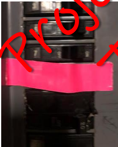
Wire exposed in at least one garden light. Circuit #9 turned off for now.
