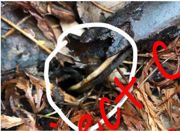
Wire exposed in at least one garden light. Circuit #9 turned off for now.
