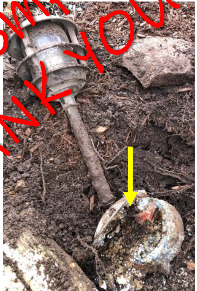
Wire exposed in at least one garden light. Circuit #9 turned off for now.
