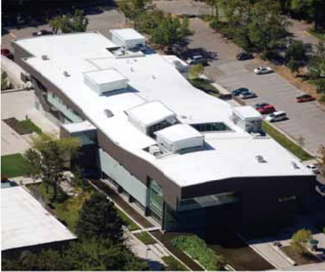
VersiFlex Roofing Systems incorporate 50-mil, 60-mil or 80-mil Polyvinyl Chloride (PVC) membranes.
