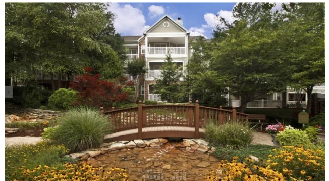
Bridges at Mallard Creek, Charlotte, NC
