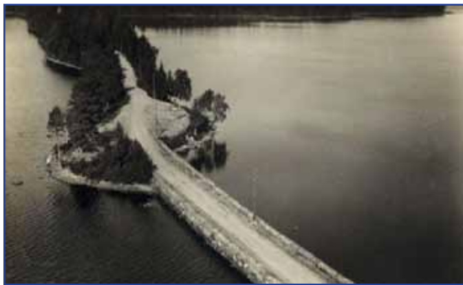
Kivisalmi Bridge facing north, circa 1937.
