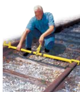
Restore Track Gauge
