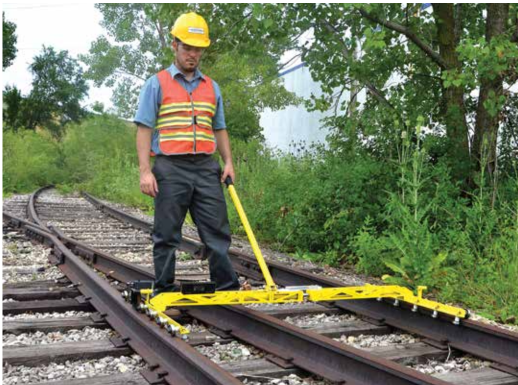
Gauge scale (55.5 - 58.5") can be read through a lexan lens from either side of Roadmaster.
