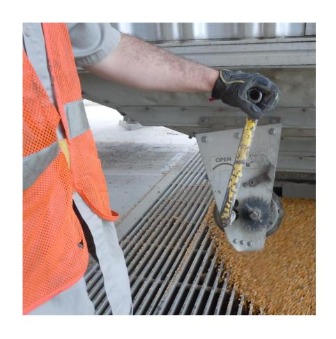
Inspect hopper gate handles prior to use looking for sharp edges, burrs, etc.
