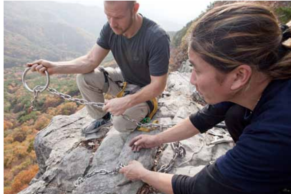
Bryan Hylenski (KOTri) and Choi Byeong Ho installing a new anchor during an initiative.
