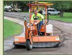
A local construction employee works diligently on the center's new paving project.
