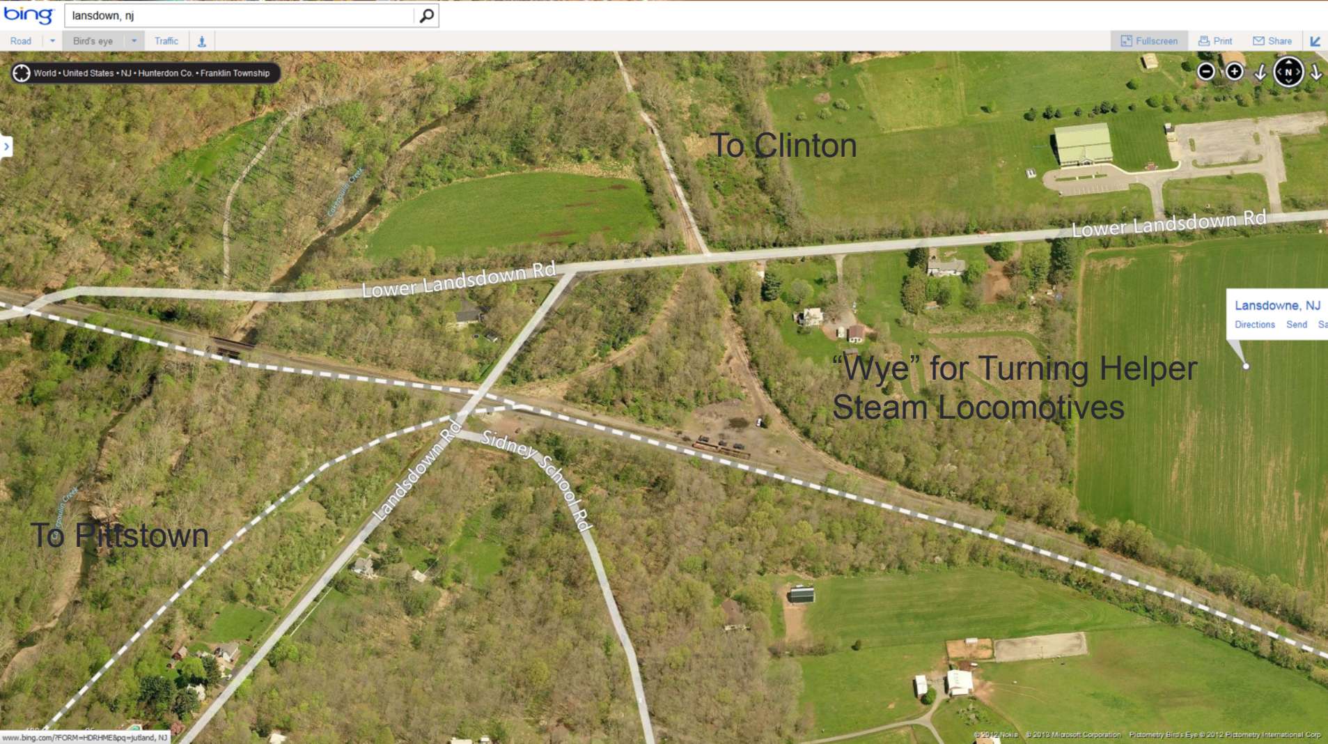
Landsdown, NJ: Steep grade west to tunnel begins here
