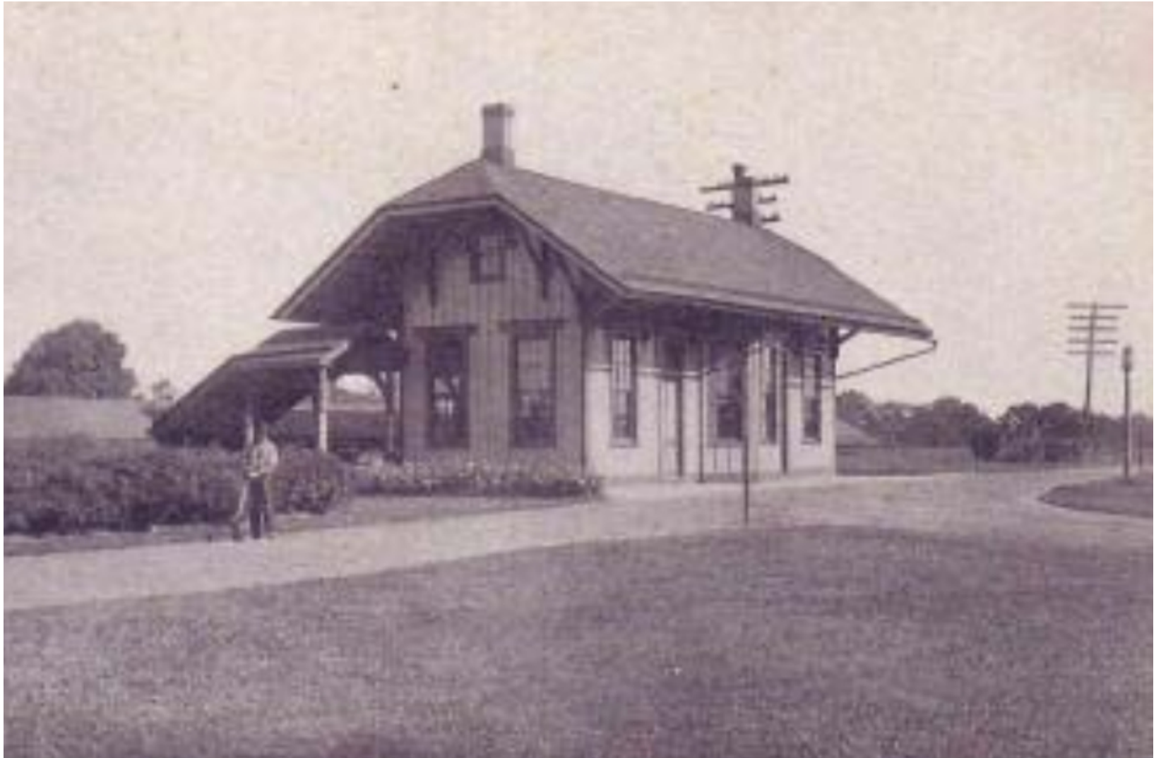
Flemington Junction Depot
