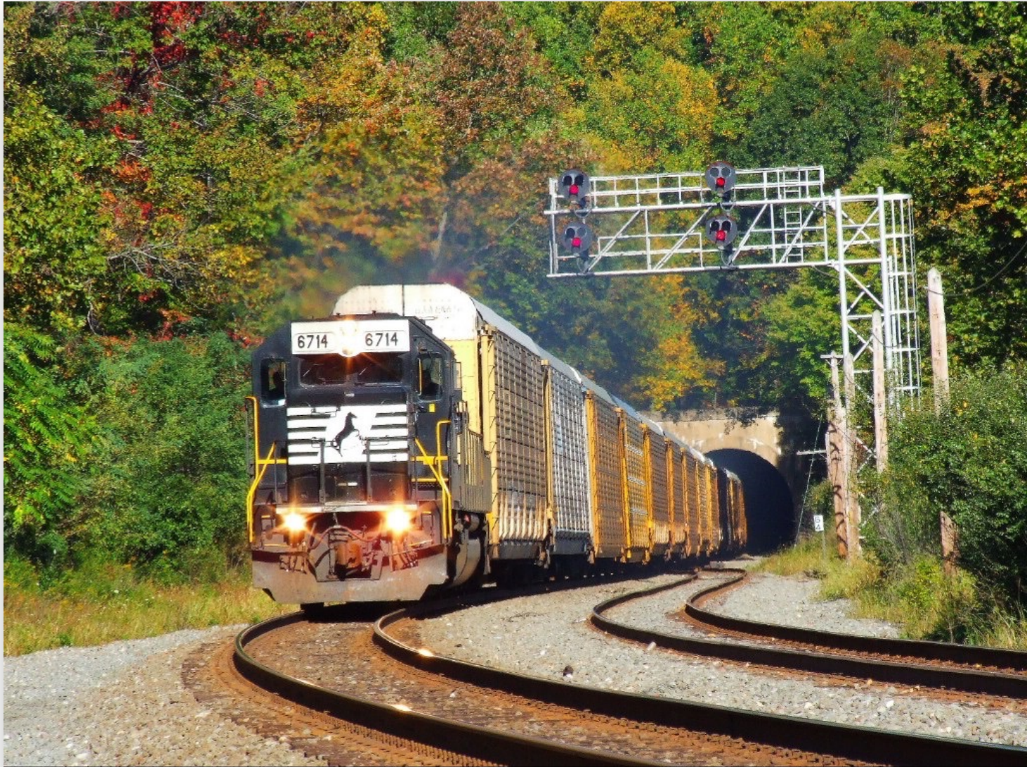
“New” Pattenburg Tunnel: Modified in 2000 for Double Stacks
