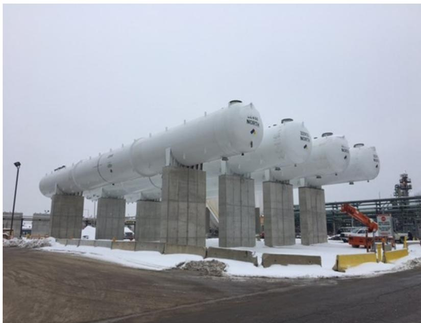
Four new liquefied petroleum gas (LPG) tanks are part of a project to move the refinery's LPG storage.
