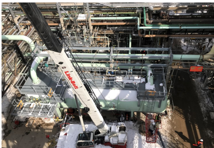
The refinery flare at Schaeffer and Dix will be removed. Above, preparations for the new flare location.
