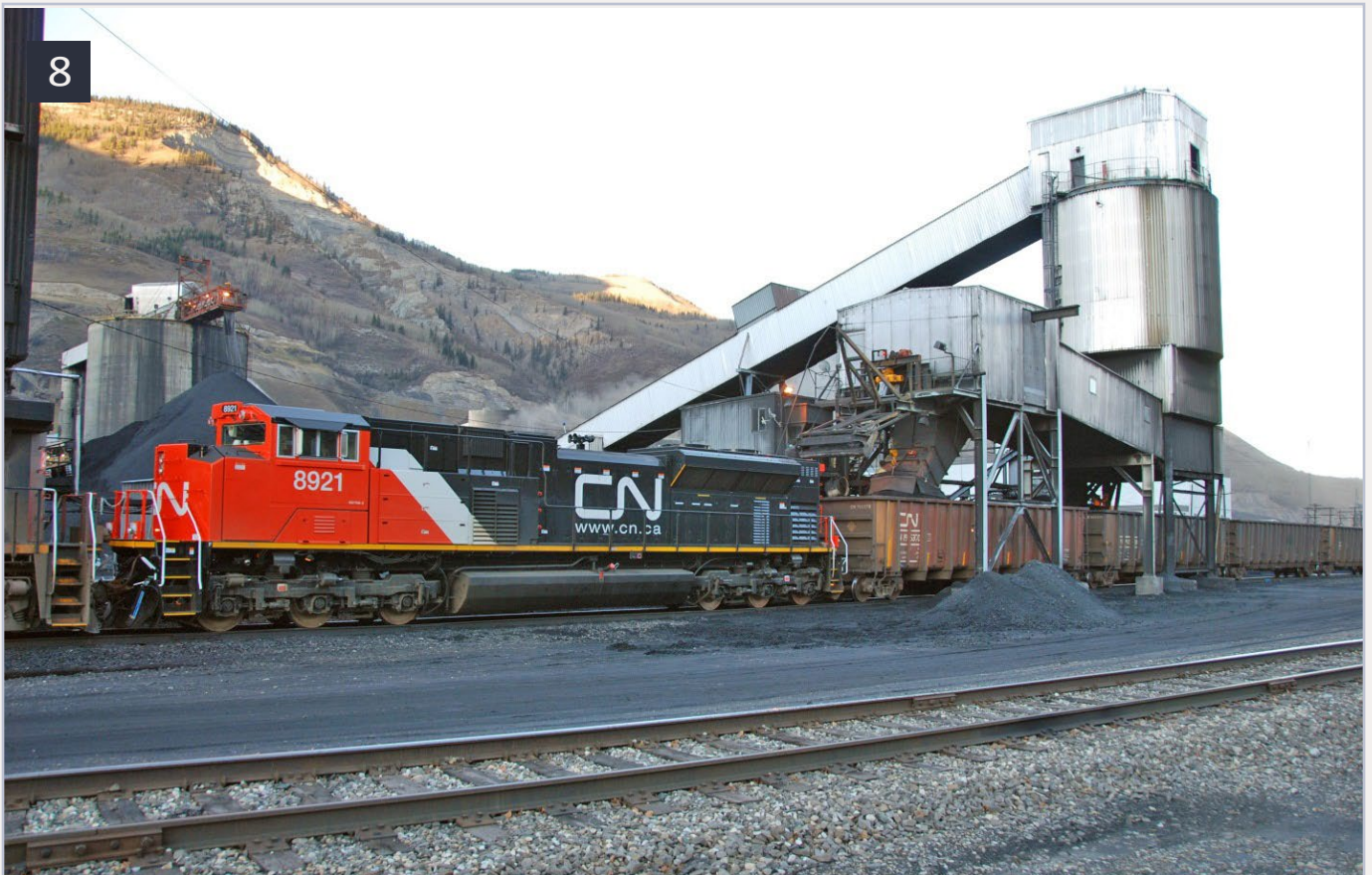
8. Coal loading facility.
