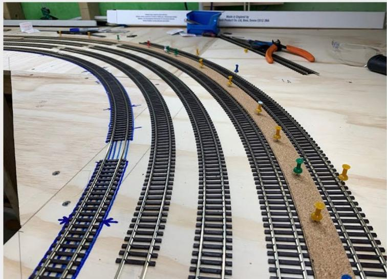
1. How do you keep the tracks parallel in a curved yard? In this thread, Jason Miller shows exactly how, along with a lot of other great hints and tips. Make sure you explore the entire thread!
