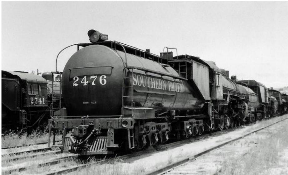
5. A unique feature for the Mayfield Branch engines was a road pilot mounted on the rear of the tenders. This modification was made because the locomotives ran backward between Los Gatos and San Jose at the end of the runs. To my knowledge, no other SP locomotives were modified in this way.
