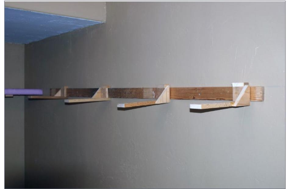
15. Gil used a method he calls “floating benchwork” to hold up the lightweight upper deck of his layout. Because the upper deck is made of extruded pink foam insulation, this simple frame nicely supports it and allows a minimal deck depth.
