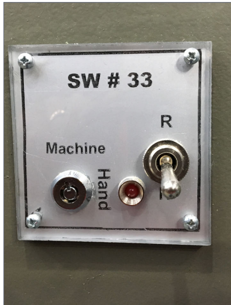
30. Switch locks and software timers can add realism and extend the duration of the run for crews.
