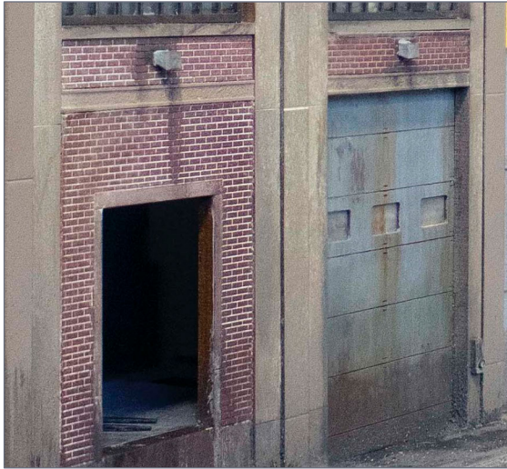
3. I added lighting over the doors as shown here.
