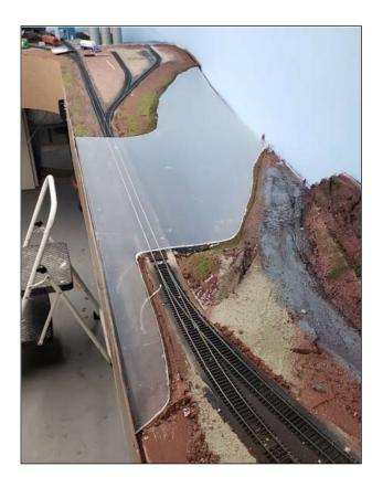
7. Test-fitting the plexiglass to make sure the lake is level.
