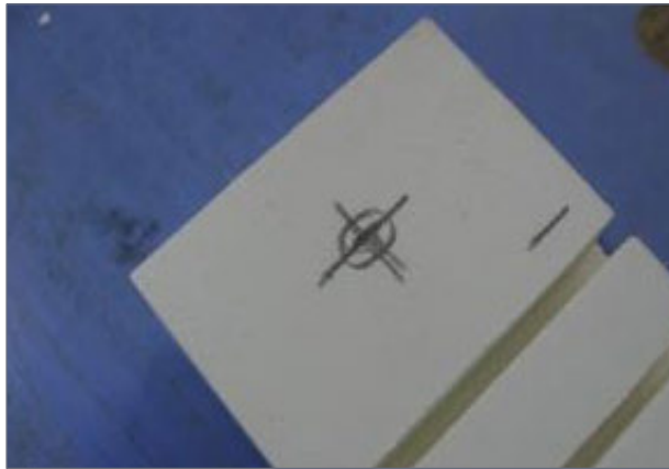
13. Mark location for mounting screw.
