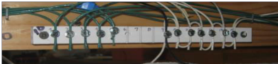
7. Serpentine common wire at right end of terminal strip.
