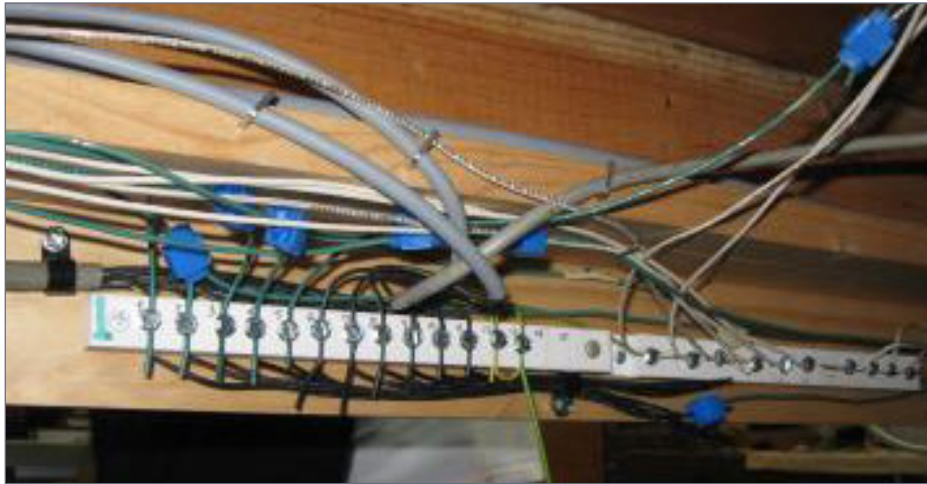
6. Narrow terminals with room for only one screw. We used suitcase connectors to add a second wire. Also on the right, notice the one long-slot common terminal strip with the white wires overlapping.
