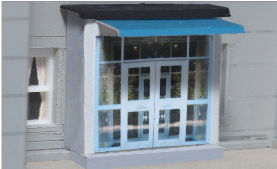
20. Aluminum vestibule for the lobby of Tanenbaum Arms. Older buildings that have been modernized often feature this type of entry.
