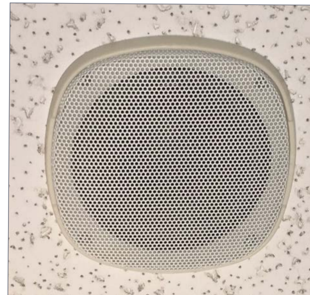
9. Ceiling speaker installation.
