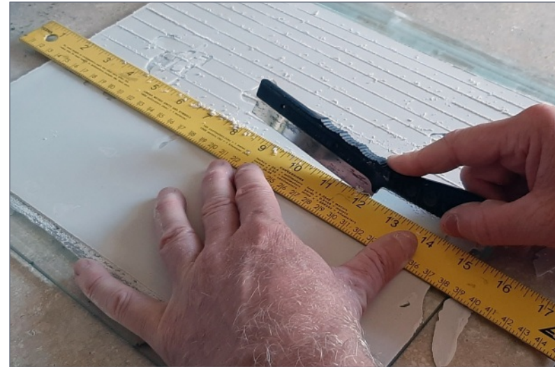
5. Scribing lines into the plaster.
