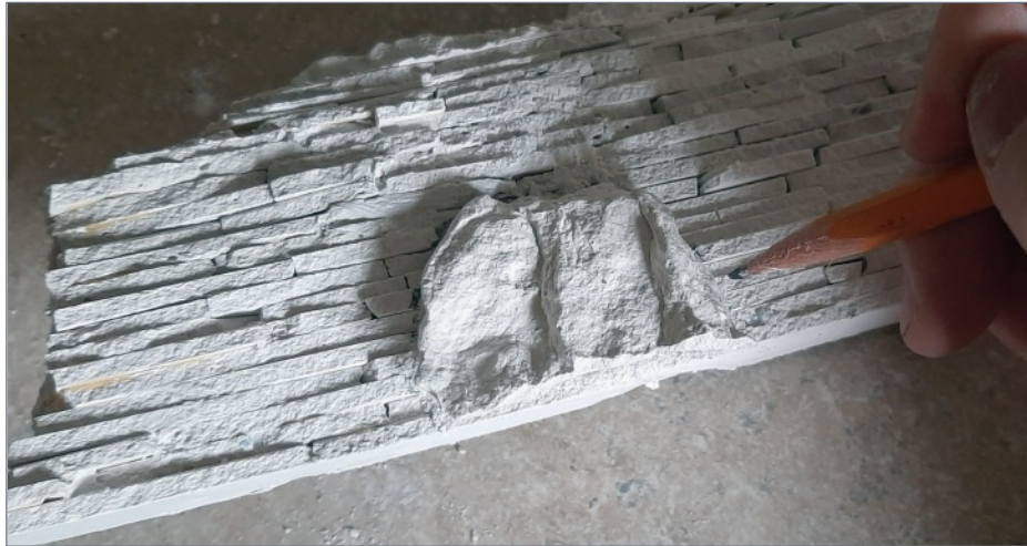
11. The outline of thin rock castings is traced onto the wall so material can be removed with a chisel blade.
