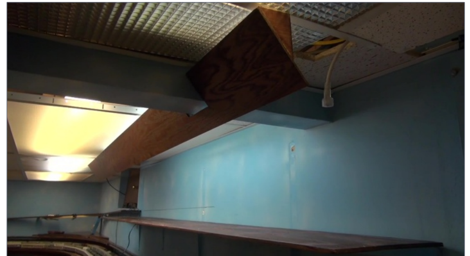
6. To add light to the shelf the module is on, Ken installs an angled valence. He'll install an LED light string later.
