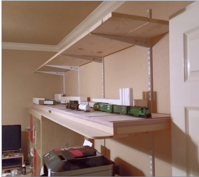
13. I added \frac{3}{4} " of foam to the top of the doors, and mounted the 10-foot shelf in place using shelf brackets. I will add a backdrop and valance overhead.
